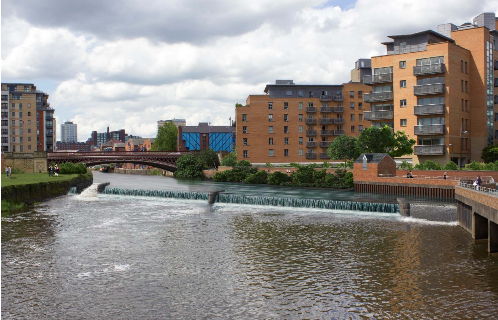
Figure 5: Downstream visual representations of masonry finishes
