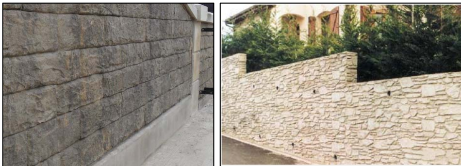
Photos 10 and 11: Pigmented Concrete with masonry imprint
